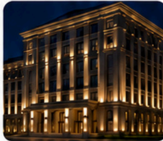
Facade Lighting Pg. 61
